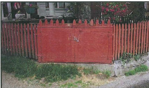
Wooden enclosure. Strengths: Secure to ground, seamless construction, directly accessible to refuse collection, and clip fastening latch.
