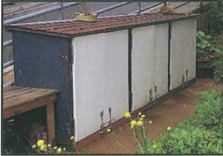
Wooden enclosure. Strengths: Heavy duty hinges and latches, seamless construction and holds six plus cans.
